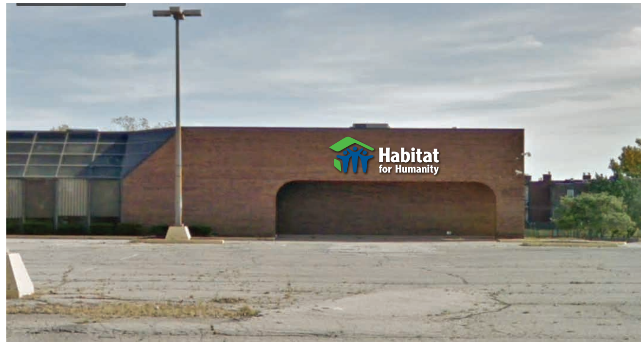
West Elevation - Office Entrance
